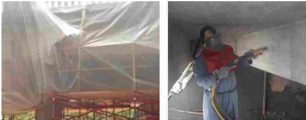
Figure 4.2. Surface Preparation by Sand Blasting
