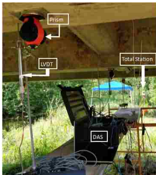
Figure 5.3. Data Acquisition System Setup
