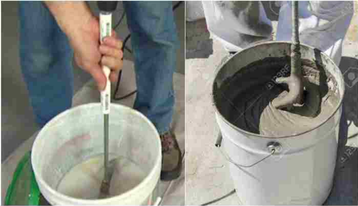
Figure 4.4. Mixing Resin and Cementitious Matrix
