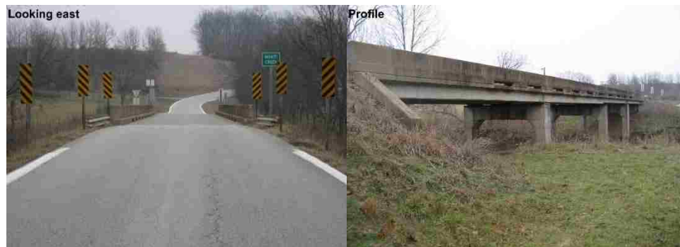
Figure 3.2. Bridge P-00585 Approach and Profile View
