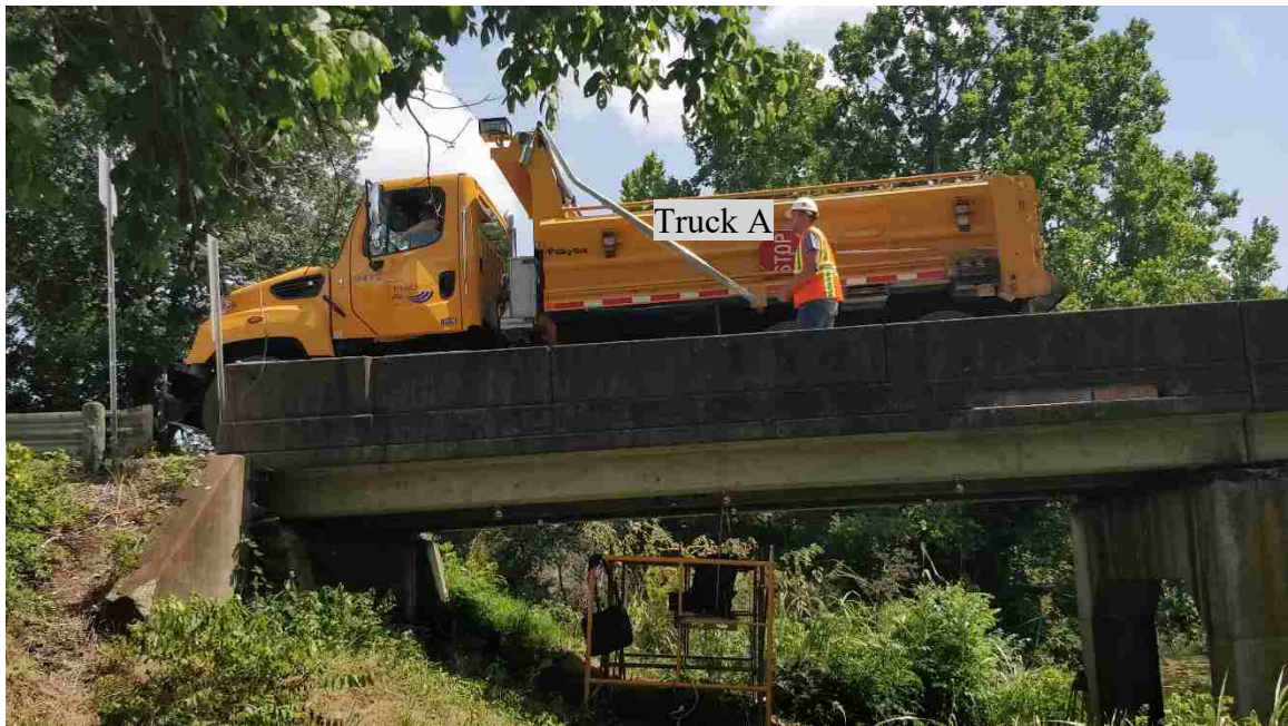
Figure 5.8. Truck on Span 4 for Load Test
